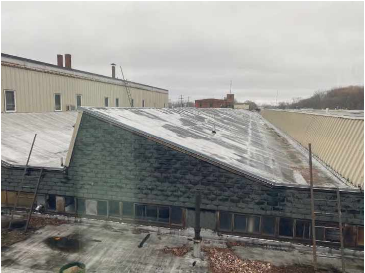
Photo 21 – Subject property roof Bldg. A (front) facing east
