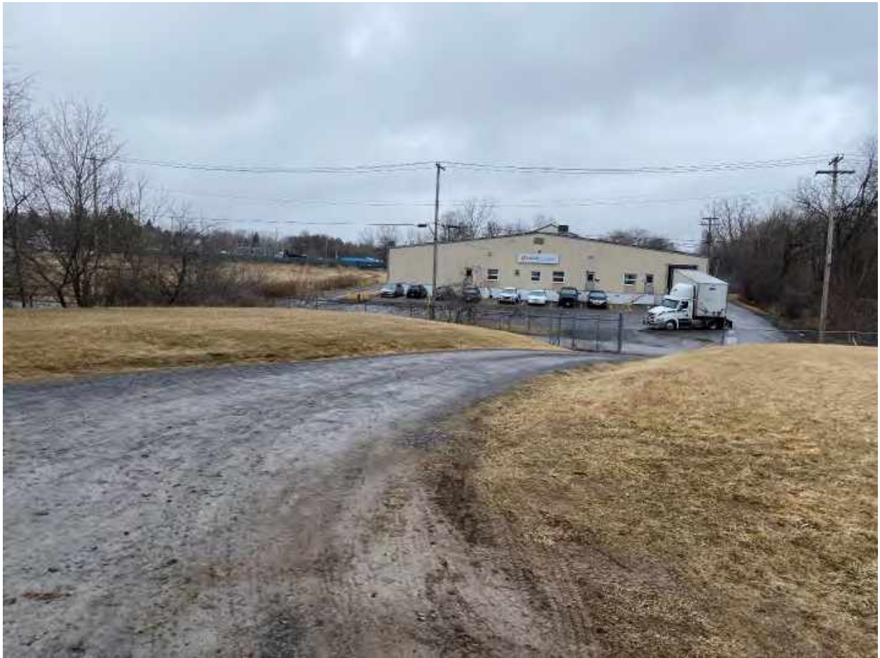
Photo 11 – Univar Solutions, former H.B. Fuller Monarch VCP Site. Facing north
