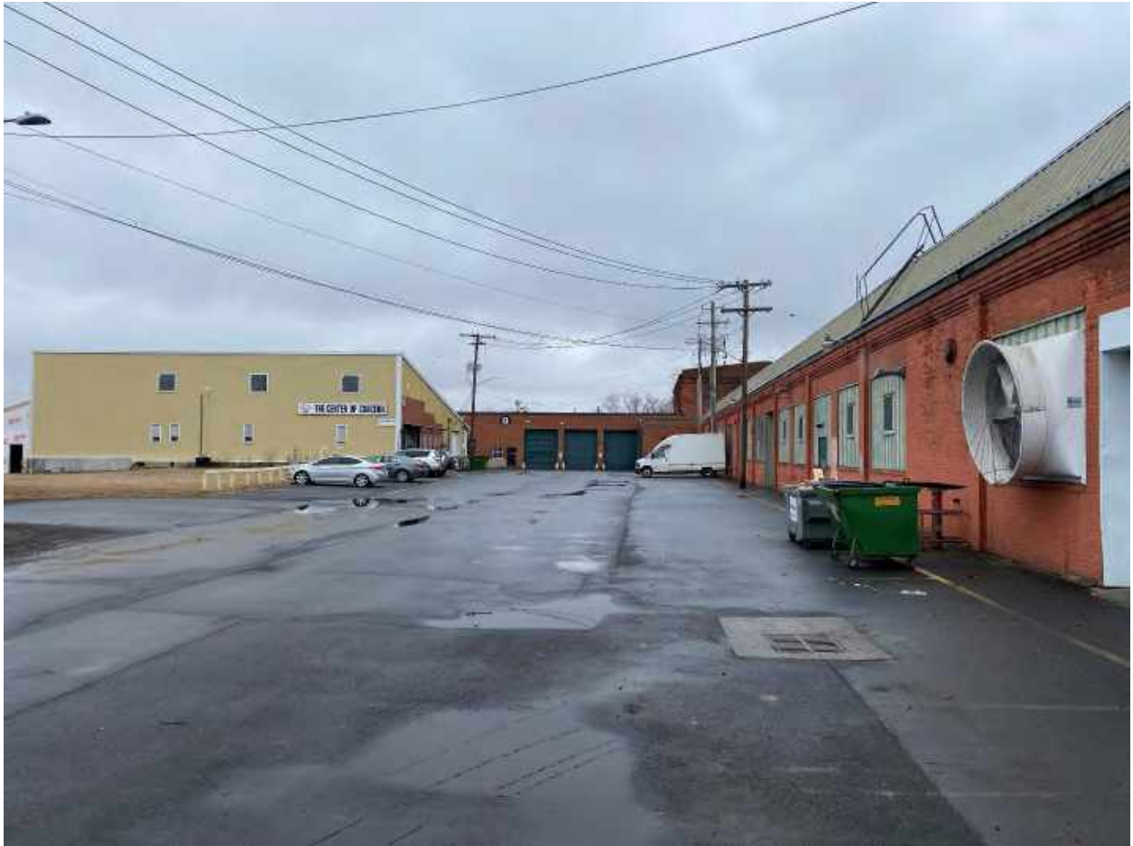
Photo 3 – Subject Property GEDC Bldg. A (single story) to the right and Bldg. B. (single story) straight ahead at the end of Avenue D. Facing east
