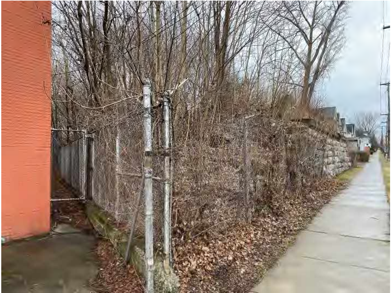
Photo 8 – Former rail embankment south of subject parcel. Sidewalk on east side of N. Genesee St. in foreground. Facing southeast
