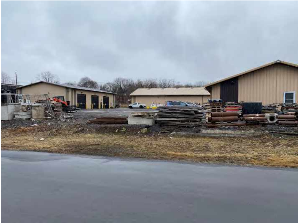
Photo 7 – Former lumber, coal and woodyard parcel. Lehigh St. in foreground. Facing west
