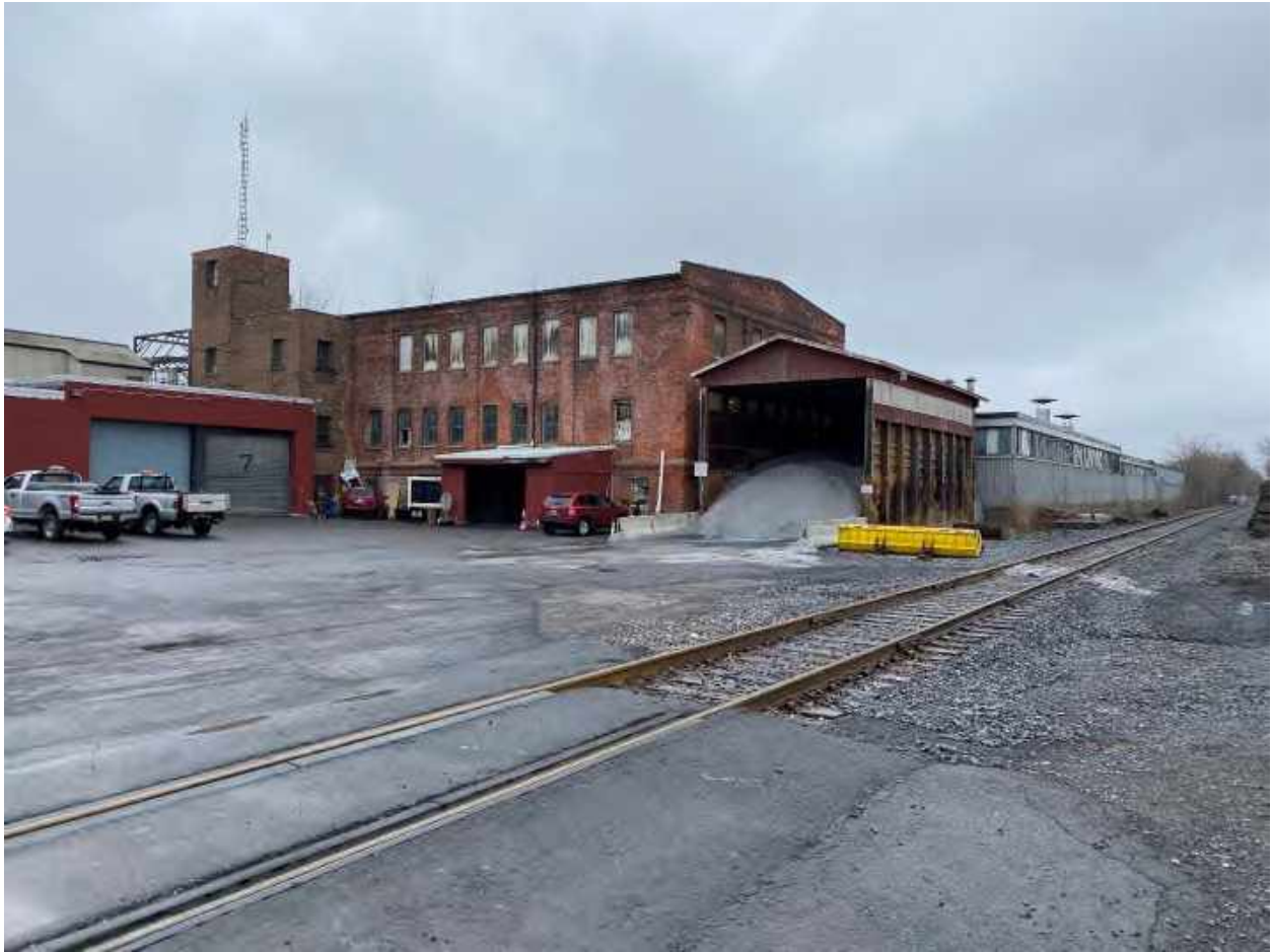
Photo 12 – Southeast corner of subject property occupied by City of Geneva DPW. Facing northwest
