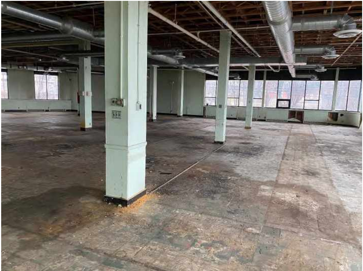
Photo 20 – Subject property second floor Bldg. A (front)
