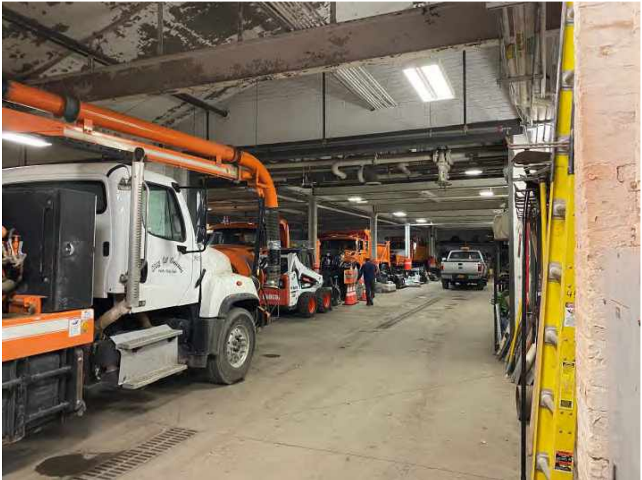
Photo 17 – Subject Property interior Geneva DPW
