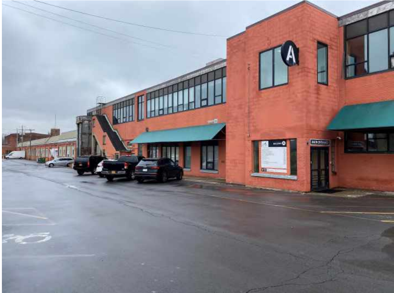
Photo 2 – Subject Property GEDC Bldg. A (2 story). Avenue D in foreground. Facing southeast
